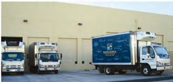
■ Santa Monica Seafood has completed construction on its new Las Vegas distribution hub.
