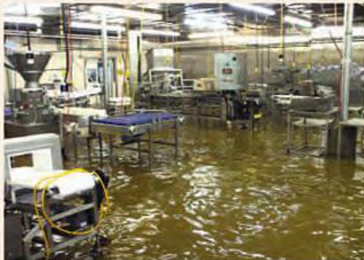
■ RICH'S PRODUCT CORPORATION plant in Gallatin, TN, is inundated by waters from heavy rains in the area on Saturday, May 1.
