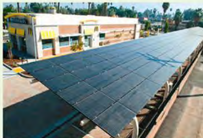
■ GOLDEN ARCHES GO GREEN - A rebuilt McDonald's restaurant in Riverside, California, has become the first McDonald's west of the Mississippi, and the fourth in the U.S., to seek LEED® Gold certification (Leadership in Energy and Environmental Design). The restaurant, located at 2242 University Avenue, opened to the public on October 14.
