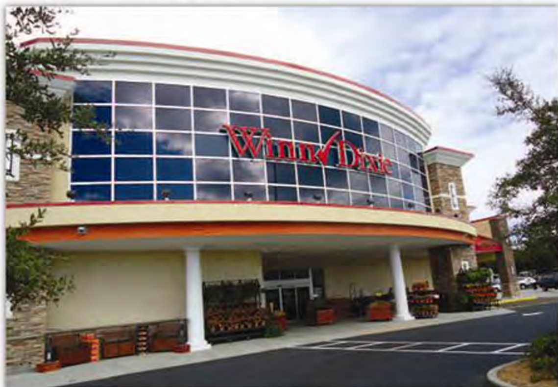
■ WINN-DIXIE'S newest transformational store opened, November 8, at 3280 S. Tamiami Trail, in the Promenades Mall plaza in Port Charlotte, Florida.
