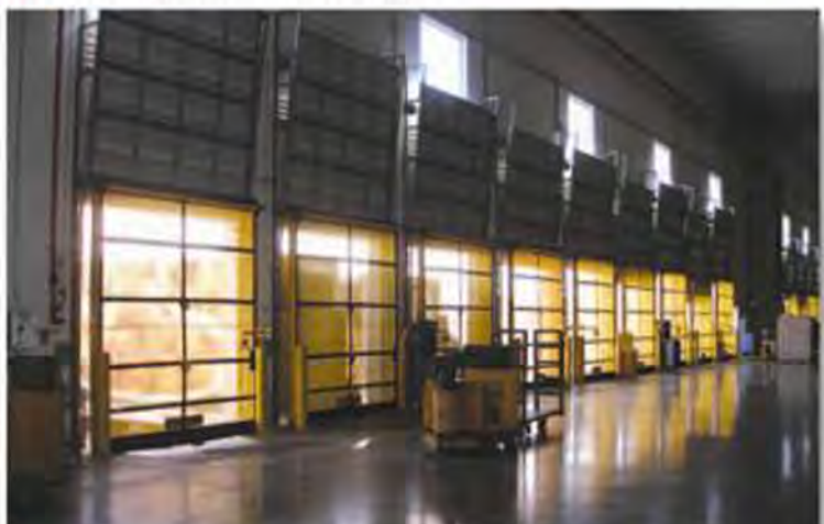
■ The new facility features 28 overhead doors with future capacity for 42 doors.
