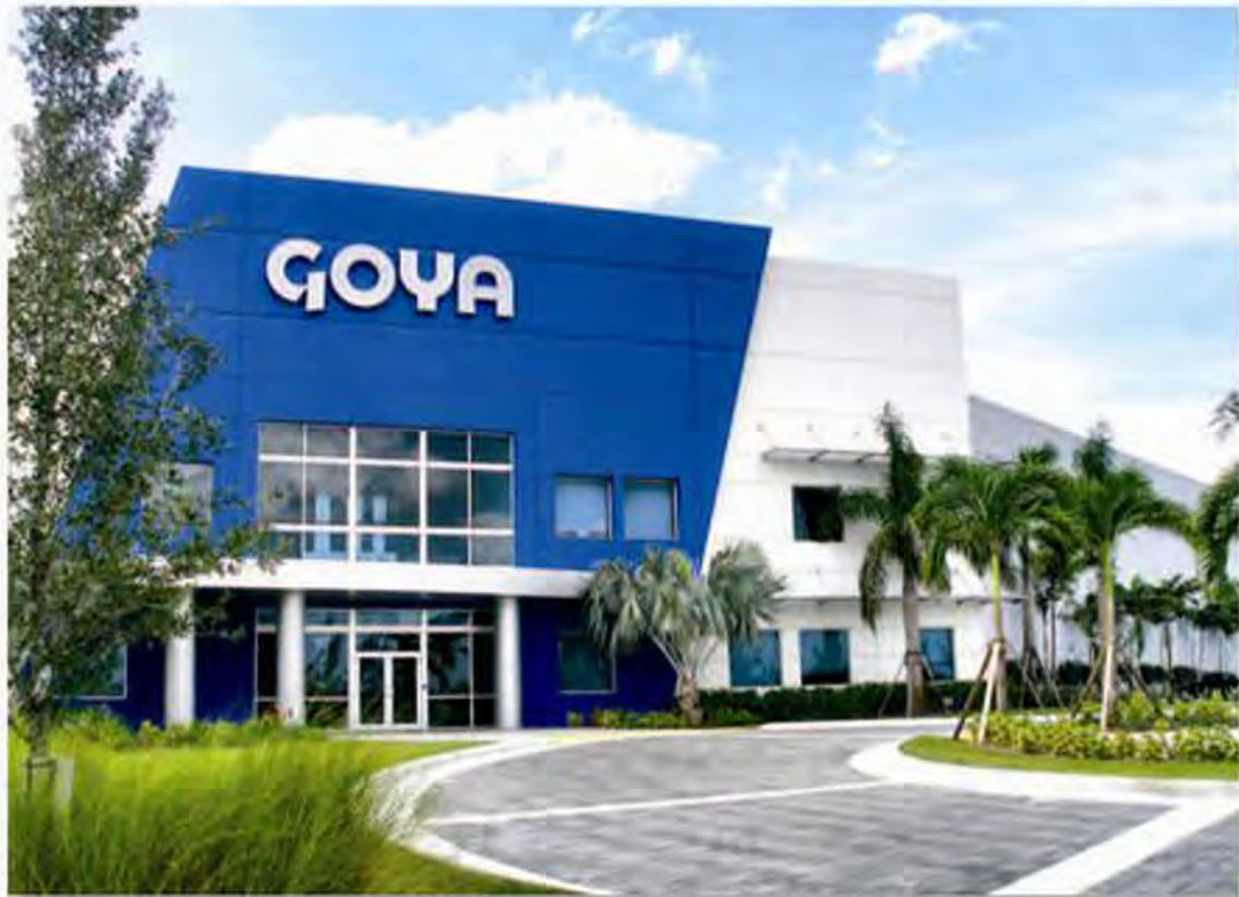
■ GOYA FOODS' new Miami Distribution Center and home of Goya Foods of Florida, is located at 13300 N.W. 25 Street in Miami. The 338,000 sq. ft. state-of-the-art distribution center which opened recently is the company's largest of its 16 facilities located throughout the United States, the Caribbean and Spain.
