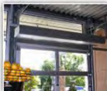
■ PRODUCE AIR CURTAINS - Air curtains are critical to Market of Choice stores because their front entrances are cost-effectively designed with automatic sliding doors versus expensive and space consuming vestibules.
