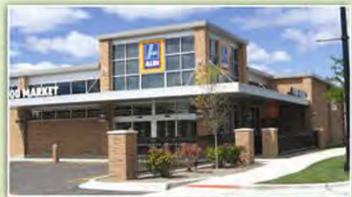
Mid-America Real Estate Corporation's Net Lease Investment Group recently announced the $1.8 million sale of a triple net ground lease for this 16,750 sq. ft. freestanding Aldi building in Chicago's south side Chatham community. The buyer is a private California investor.
