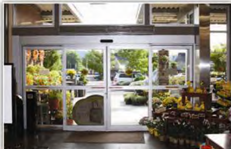
■ MAIN ENTRANCE AIR CURTAIN - Most stores use an aesthetic stainless steel Zephyr or MaxAir model air curtain manufactured by Berner International, New Castle, PA, to match the modern interior automatic door entrances.
