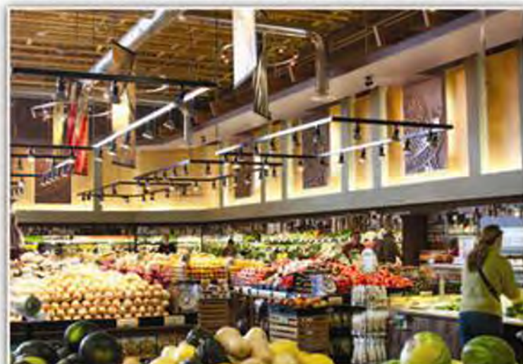
■ PRODUCE LIGHTING - Besides air curtains, another major energy conservation program is Market of Choice's transition from HID and fluorescent light bulbs to more efficient LED lighting in produce sections and reach-in coolers/freezers.
