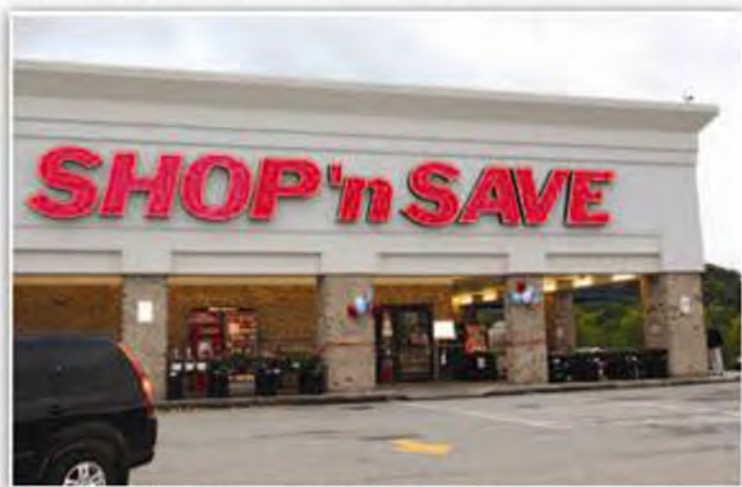
■ The top to bottom store remodel took almost two years to complete.
