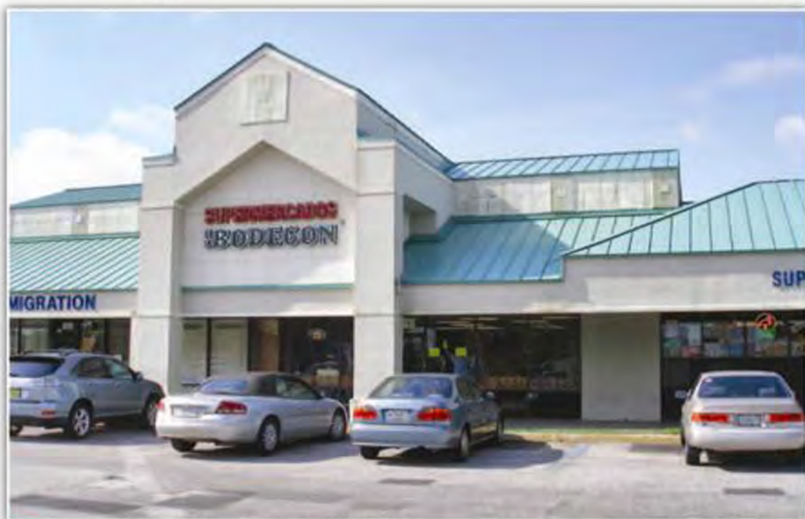
■ The expansion of El Bodegon #3, 8022 W. Sample Rd., in Margate, FL is well underway following the recent celebration of the completion of construction Phase I.
