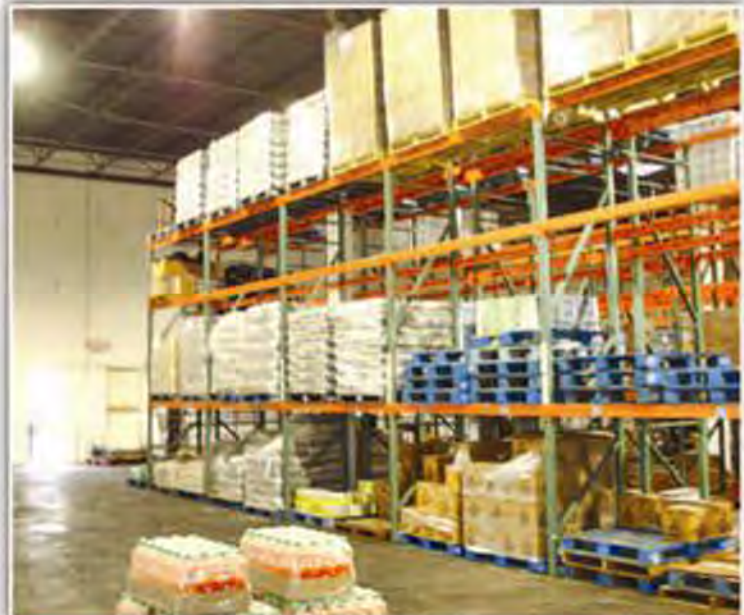
■ UNIFIED WHOLESALE GROCERS services customers from this state-of-the-art distribution center in Fort Lauderdale, Florida. The facility is conveniently situated near the airport, seaport and major highways.
