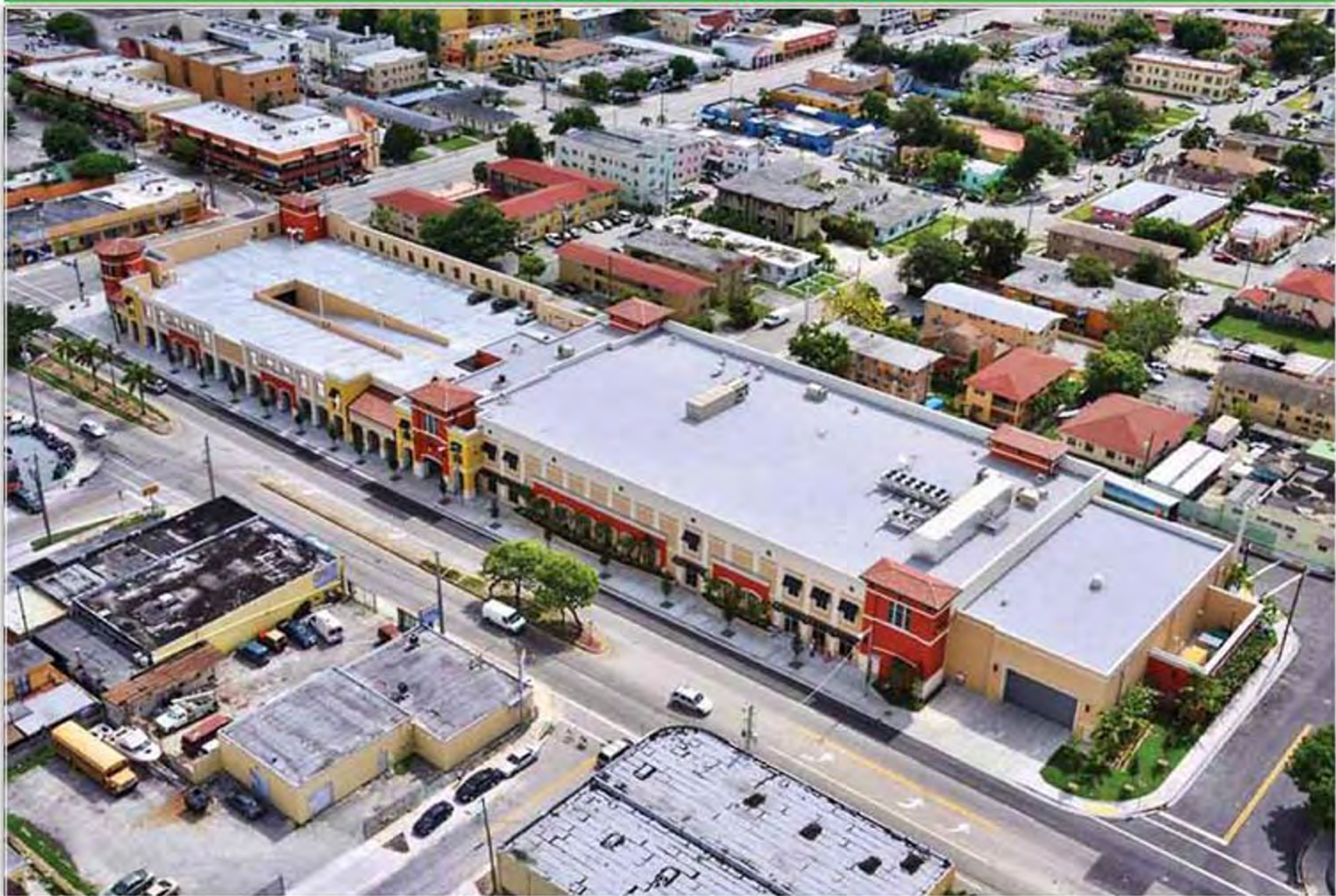
FRONT VIEW of new 28,000 sq. ft. Publix Sabor at Altos Plaza which opened in Miami's Little Havana on July 11. The two level parking garage can be viewed at the left. The supermarket is located on the right portion of the two block parcel. (Photo courtesy: Publix Super Markets/Aerial Photography, Inc.)
