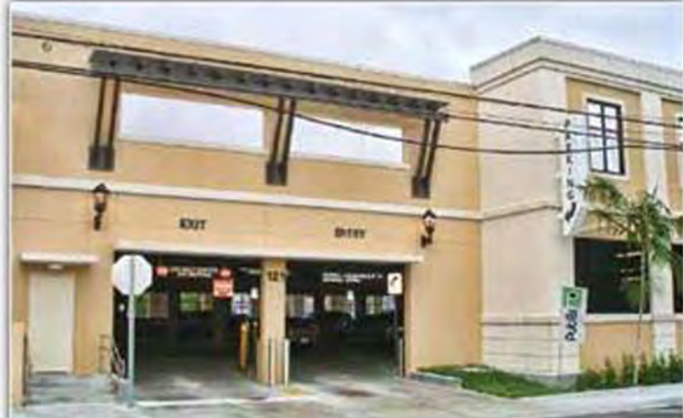
■ Entrance and interior views of the two level parking garage.
