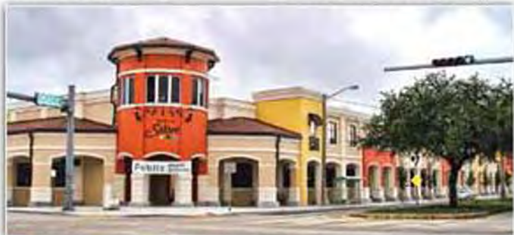
DISTINCTIVE ARCHITECTURAL APPOINTMENTS such as the cupola found at the north end of the parking garage highlight the entire structure's design.
