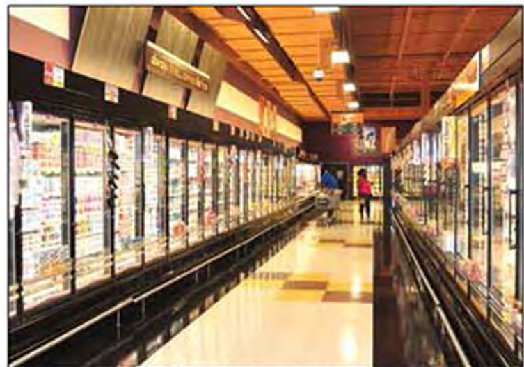
■ The ShopRite of Four Seasons Plaza was built with the latest energy-saving and sustainable technologies in refrigeration and lighting, including glass doors on the dairy and freezer cases, LED and T-8 lighting and environmentally-friendly refrigerant systems.
