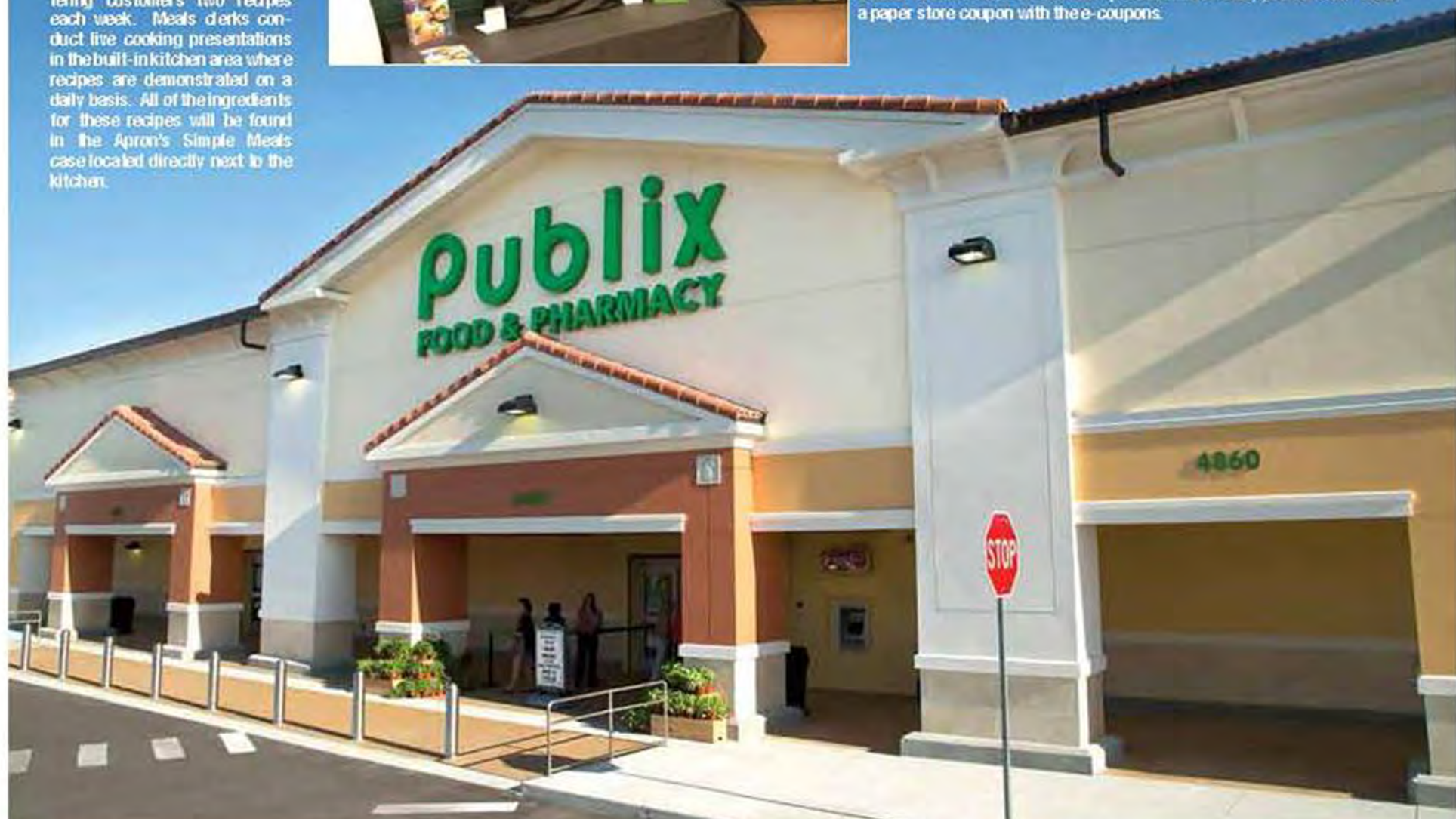
■ PUBLIX DEBUTED its newly-reopened Store #1458 at Kings Lake Square shopping center in East Naples on Thursday, April 24, after undergoing a total rebuild over the last nine months.
