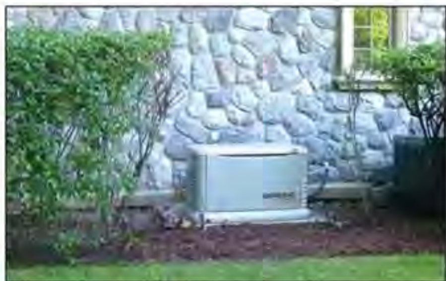
■ The 22 kW Guardian Series is the largest air-cooled home standby generator on the market. It generates enough electricity to power a smaller sized c-store or business.
